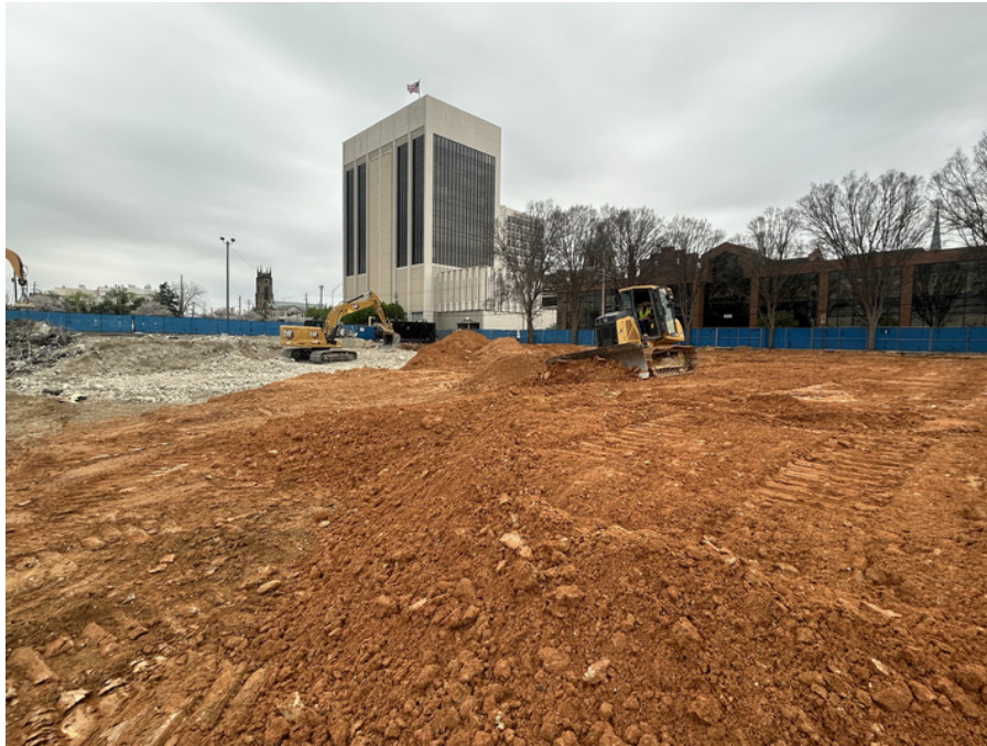
(P1) Placing fill.
