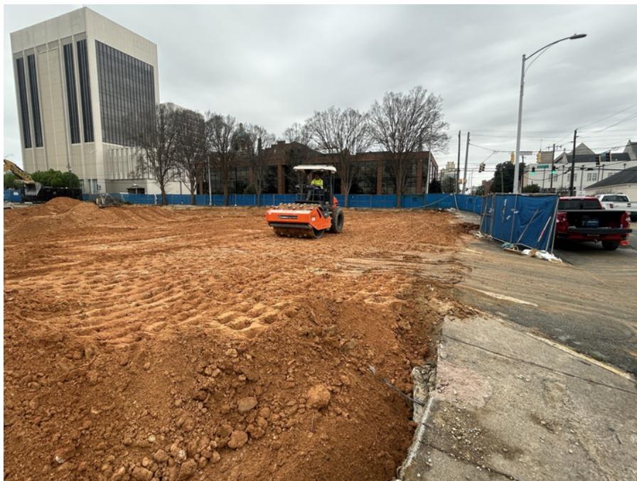
(P2) Compacting fill.
