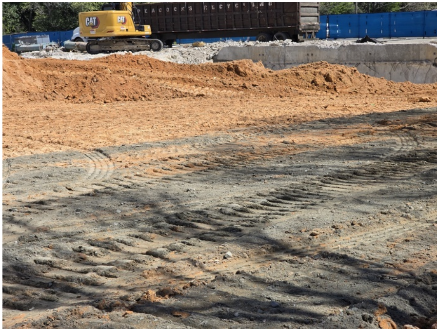
(P2) Area fill was placed
