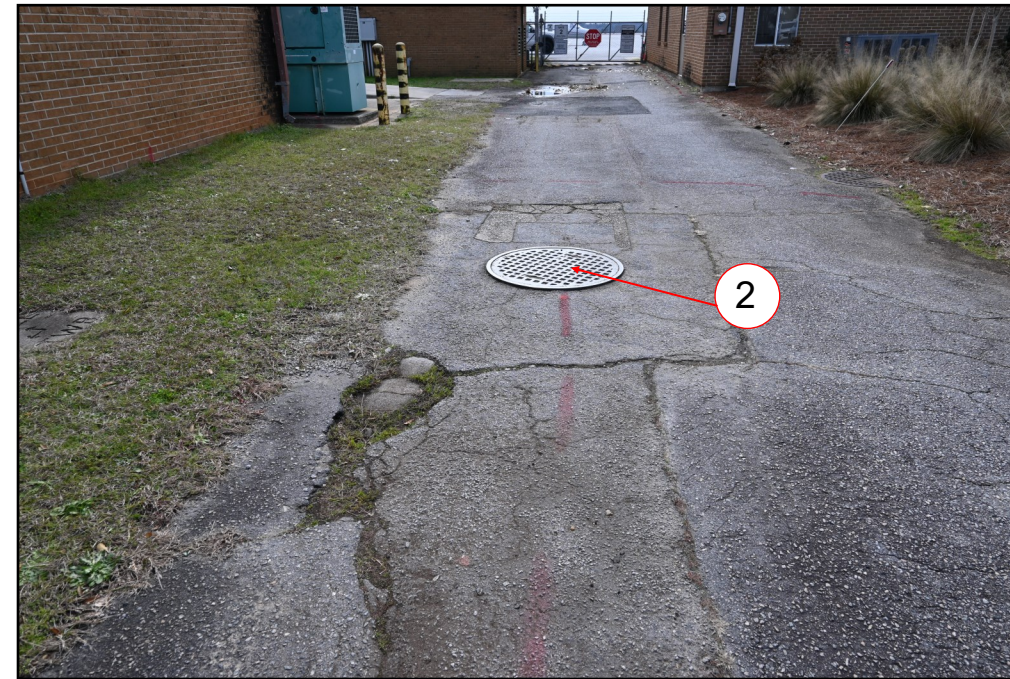
Figure 2: Electrical junction structure adjacent to Airfield Lighting Vault
