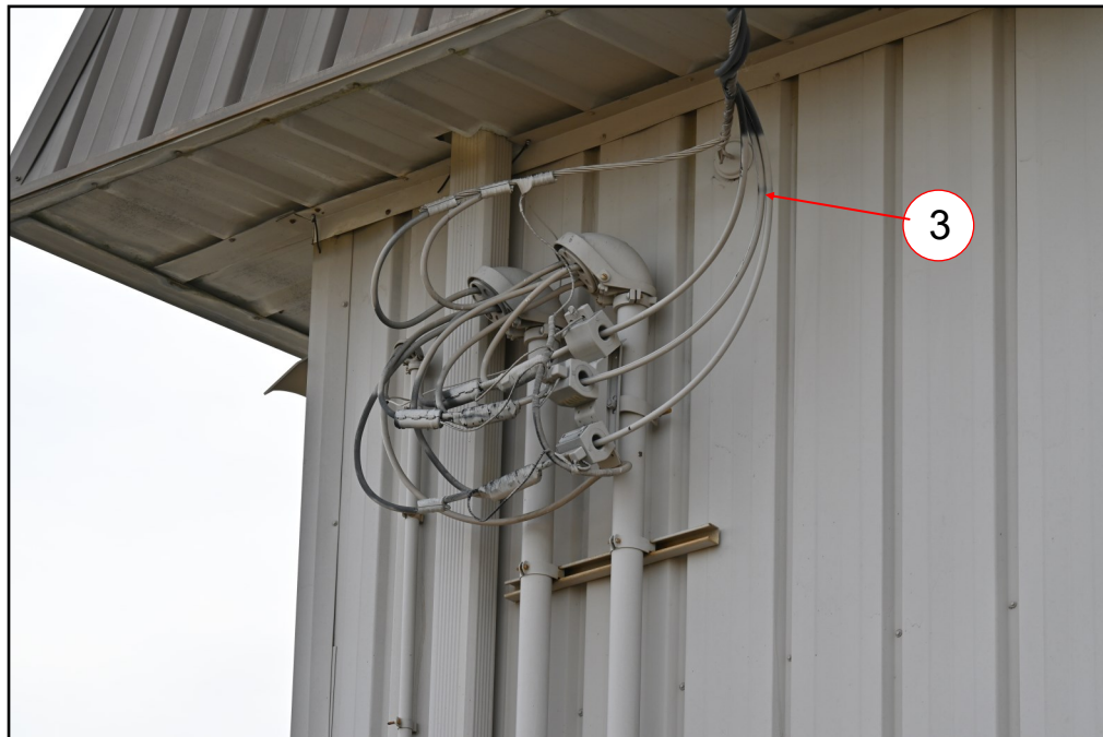
Figure 3: Twin 200 Amp, 208/120 Volt feeders to Existing FBO Terminal Building panel boards
