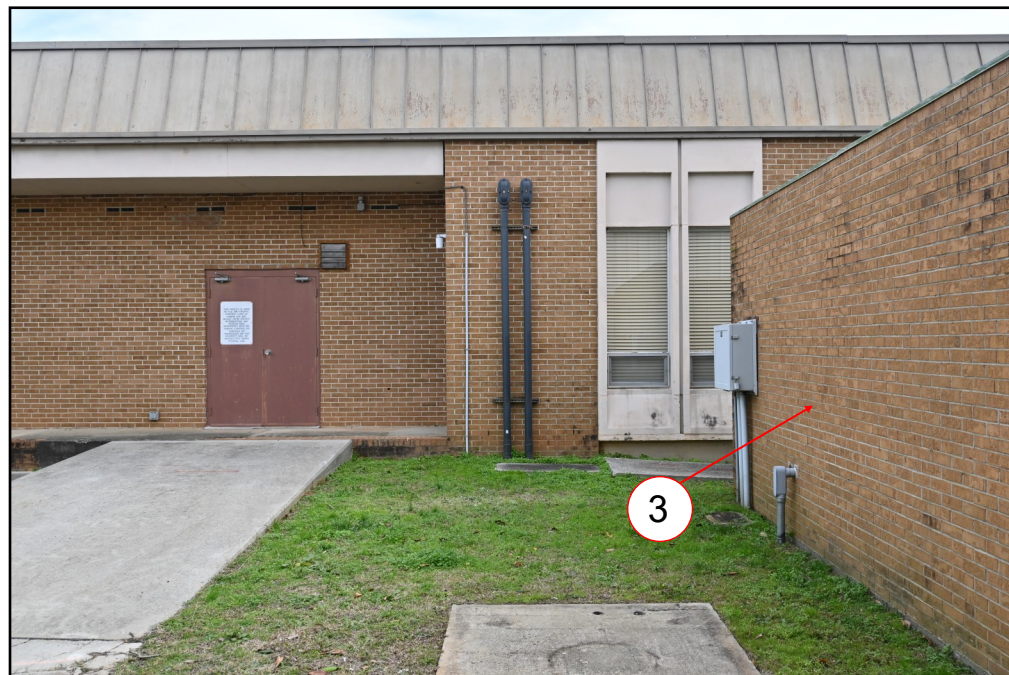
Figure 3: West view of FAA Generator Building
