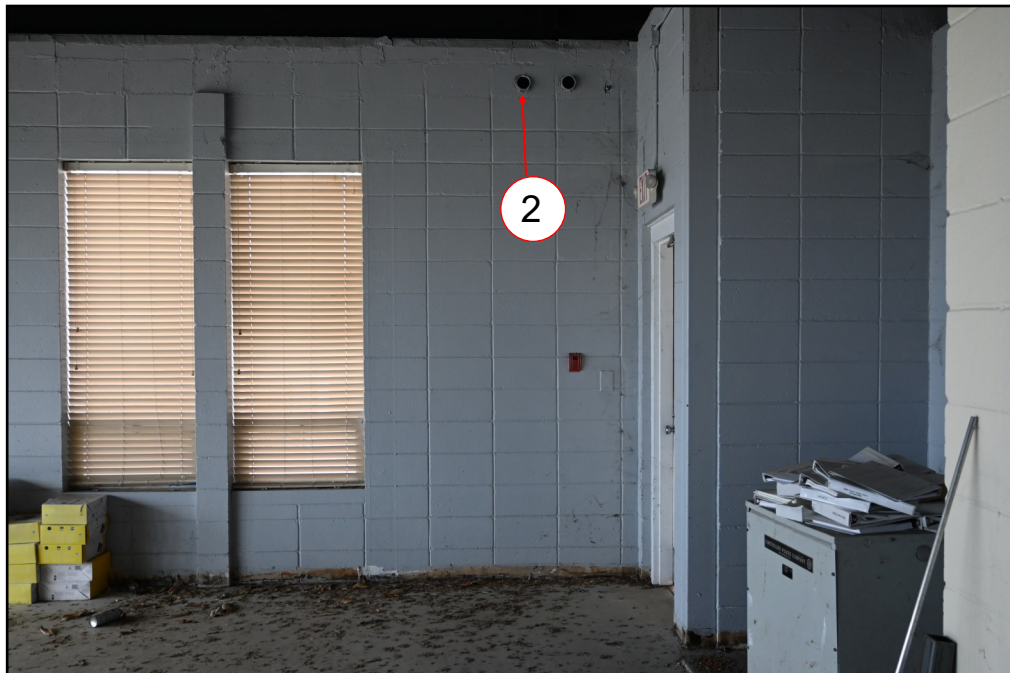
Figure 3: Termination of twin 2" PVC conduits (abandoned) in FAA Avionics Building from conduits mounted on west wall of FAA Avionics Building
