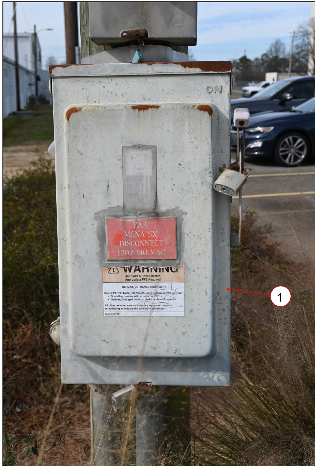
Figure 1: FAA MCNA SX Disconnect Switch 120/240 Volts in front of Existing FBO Terminal Building
