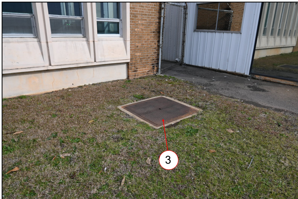
Figure 3: Airfield Lighting Ductbank junction structure at south side of FAA Avionics Building
