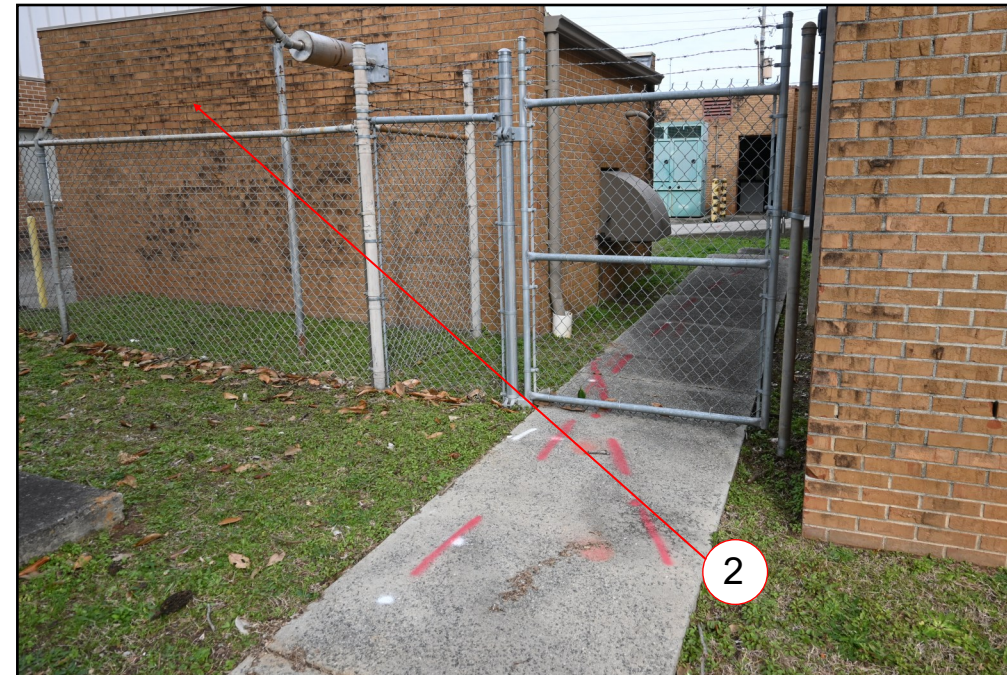
Figure 2: Southeast view of FAA Generator Building
