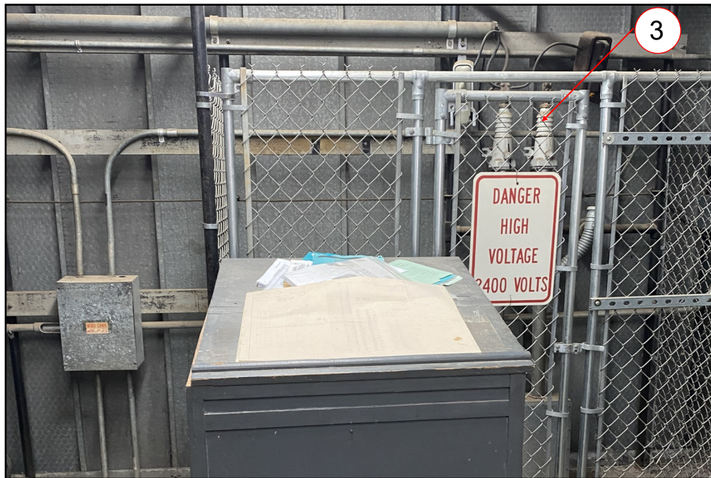
Figure 3: Airfield Lighting Vault incoming power transformer 1 of 2 (2400 Volt primary, 240 Volt secondary)
