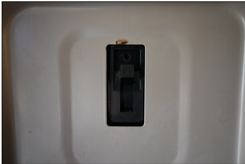
Figure 3: 200 Amp, 3 pole main circuit breaker for panel board 2 of 2 in existing FBO terminal Building
