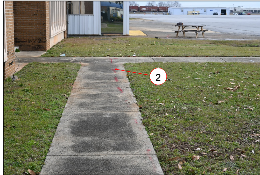
Figure 2: West to East view of Airfield Lighting Ductbank
