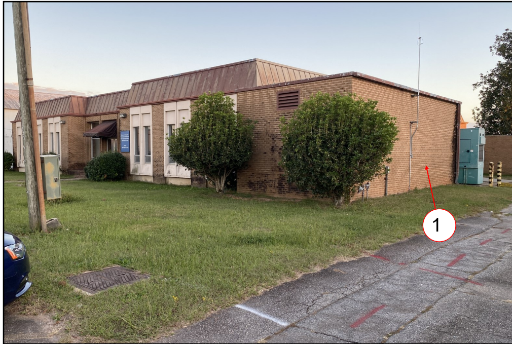
Figure 1: Airfield Electrical Vault at west side of FAA Avionics Building
