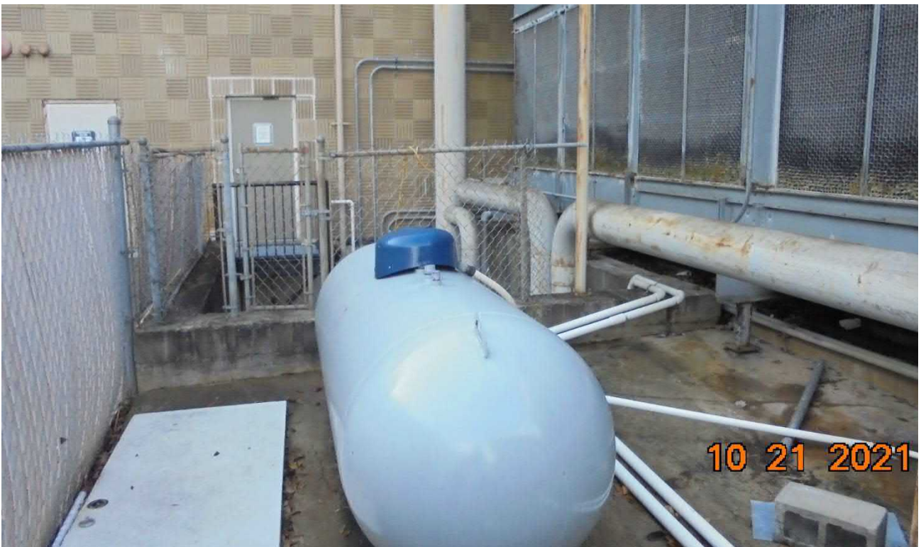
Photo 8: View of propane AST located on the northwest side of the subject building
