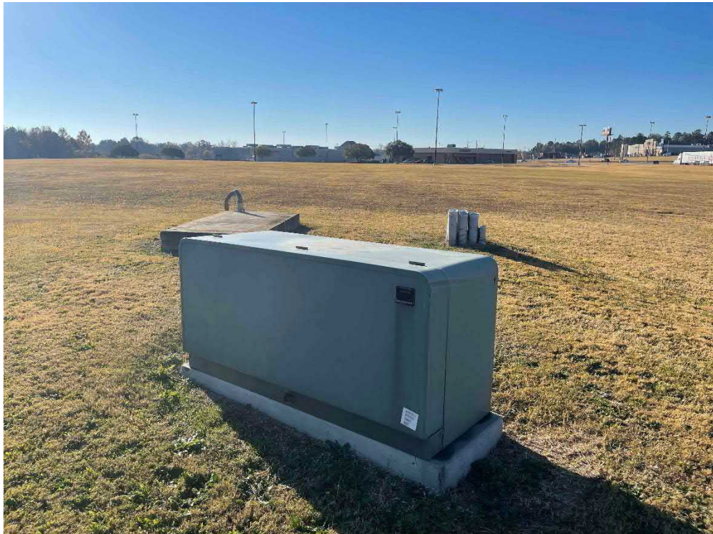
Photo 14: View of pad-mounted transformer and wastewater lift station within the northeastern portion of the site
