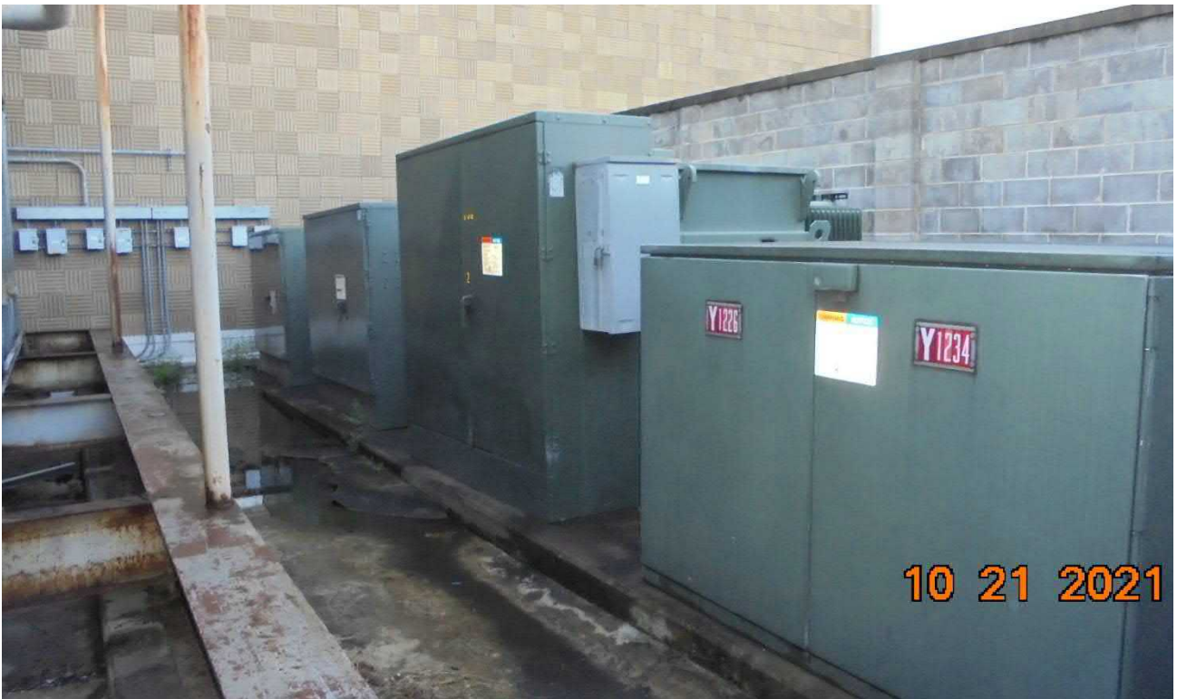
Photo 9: View of pad-mounted transformers located on the northwest side of the subject building
