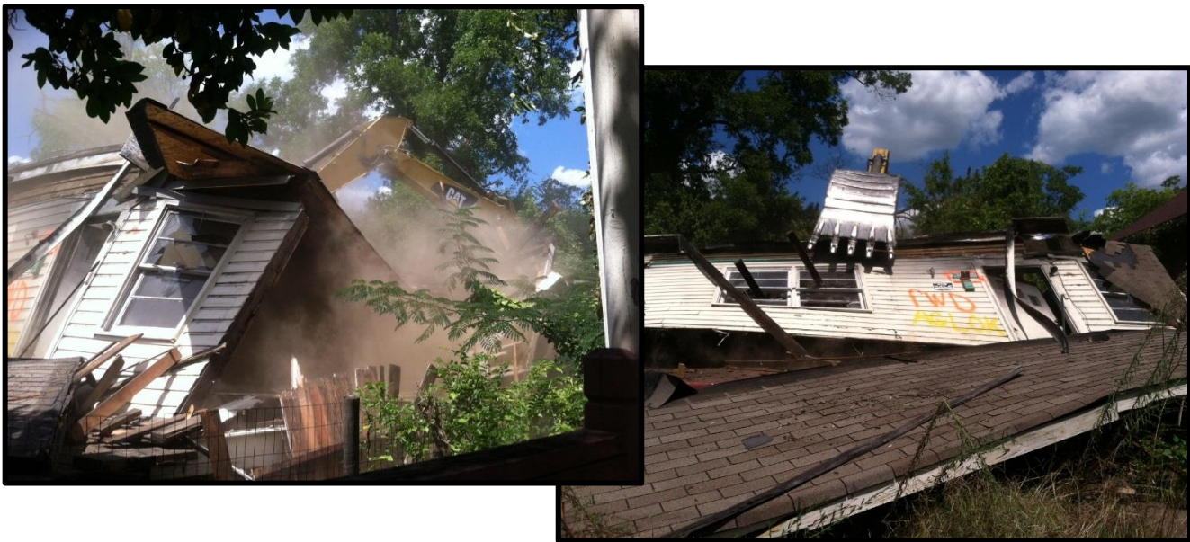
Demolition of Blighted Structure
